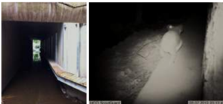
Figure 2: The left hand panel shows the design and layout of a ‘safe passage’ under a major road. Note the raised animal walkway on the right hand side of the tunnel. The Right hand side panel (infrared image) shows a koala using the raised walkway through this tunnel to safely move from one side of the road to the other at night.
